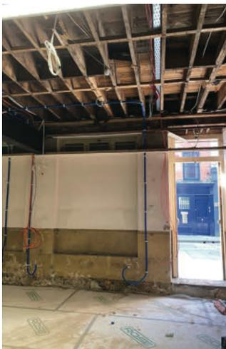
was taken. This revealed nearly 18 inches of extra head room once various services were accommodated. The opportunity to enhance the ventilation system, to bring the electrical and fire detection systems into compliance with current health and safety requirements and to install state of the art lighting with audio visual capability was greatly welcomed.
